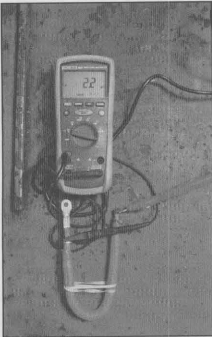
Test HV cables for shorts to ground using a MegOhm meter.
